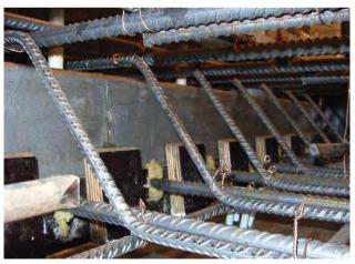
Figure A.10 Picture of the formwork where the rebars crosses the injection channels.
