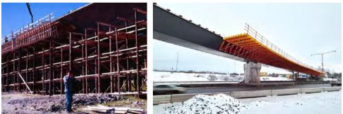
Figure 2.1 One concrete bridge and one composite bridge under construction.
