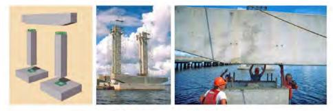
Fig. 6. Prefabricated substructures (FHWA 2009)
