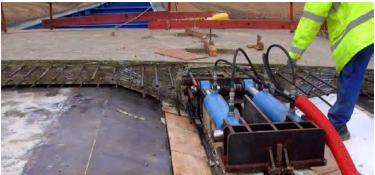
Figure 2.9 Launching of the first segment (Berthellemy 2009).
