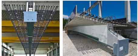
Figure 2.5 VFT-girder at different production stages (Seidl 2009b).
