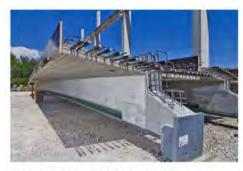
Fig. 8. Prefabricated VFT-girder (Reprinted with permission from Seidl and Braun 2009) in the longitudinal direction of the bridge. The concrete deck on top of the upper flange of the box girder is also cast in place.
