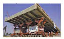
Fig. 4. SPMT transportation of 4500 South Bridge, Utah (Reprinted with permission from Manunoet USA South, Inc.)
