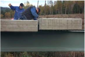
Figure 7.4 Erection of deck elements.
