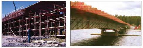
Fig. 1: One concrete bridge and one composite bridge during construction
