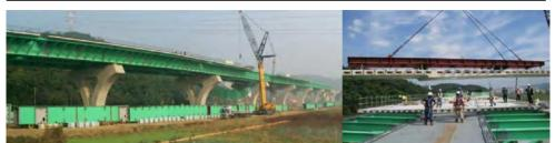
Figure 2.4 Erection of deck panels on the Secheon Bridge (Shim et al. 2010).
